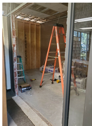
New Meeting Room Under Construction
